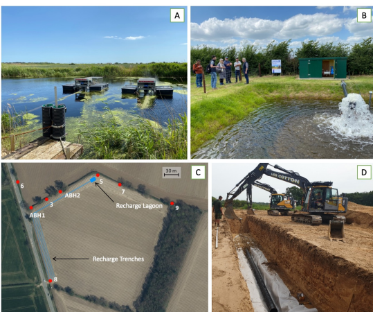
Fig. 2 A: Surface water abstraction location in the King's Fleet showing the eel-friendly, Riverscreen source-water pumps. B: Recharge lagoon at the Bucklesham MAR site in operation. C: Abstraction borehole (ABH1, ABH2) and observation borehole location plan, including the position of the recharge lagoon and layout of infiltration trenches. D: Recharge distribution trench under construction.
