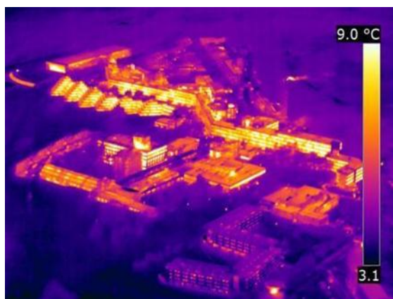
Fig 12. Infra-red aerial image of UEA campus taken in January 2011: This clearly illustrates the long term challenge of our 1960's buildings, and the importance of our programme of long term improvement.
