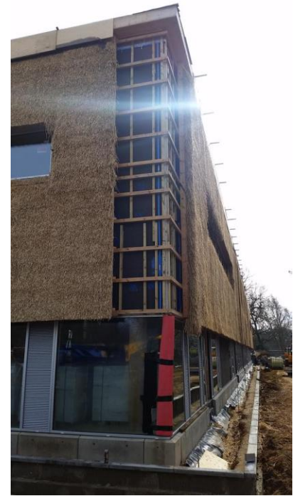
The installation of highly innovative thatched cassettes cladding is a world construction first
