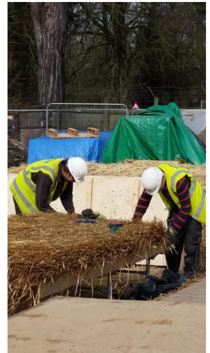
The installation of highly innovative thatched cassettes cladding is a world construction first
